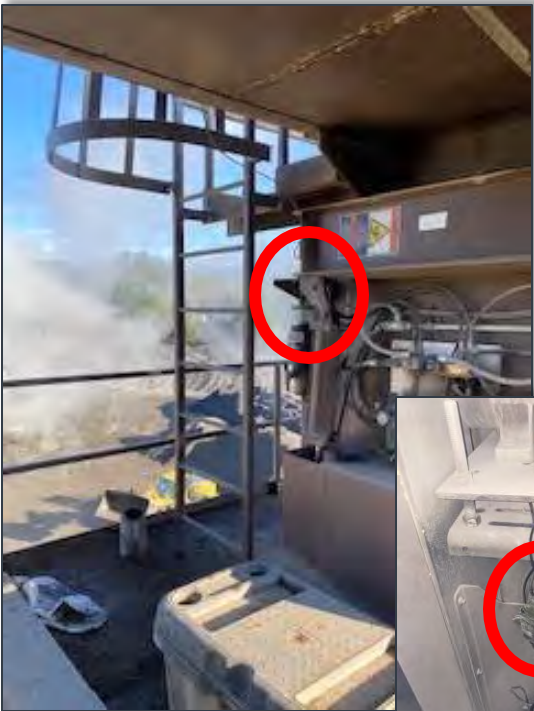
One particulate analyzer placed at the top of the silo
