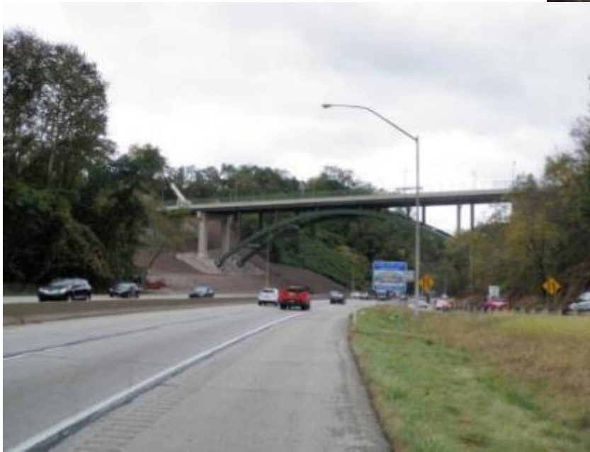
Greenfield Ave Bridge City of Pittsburgh
