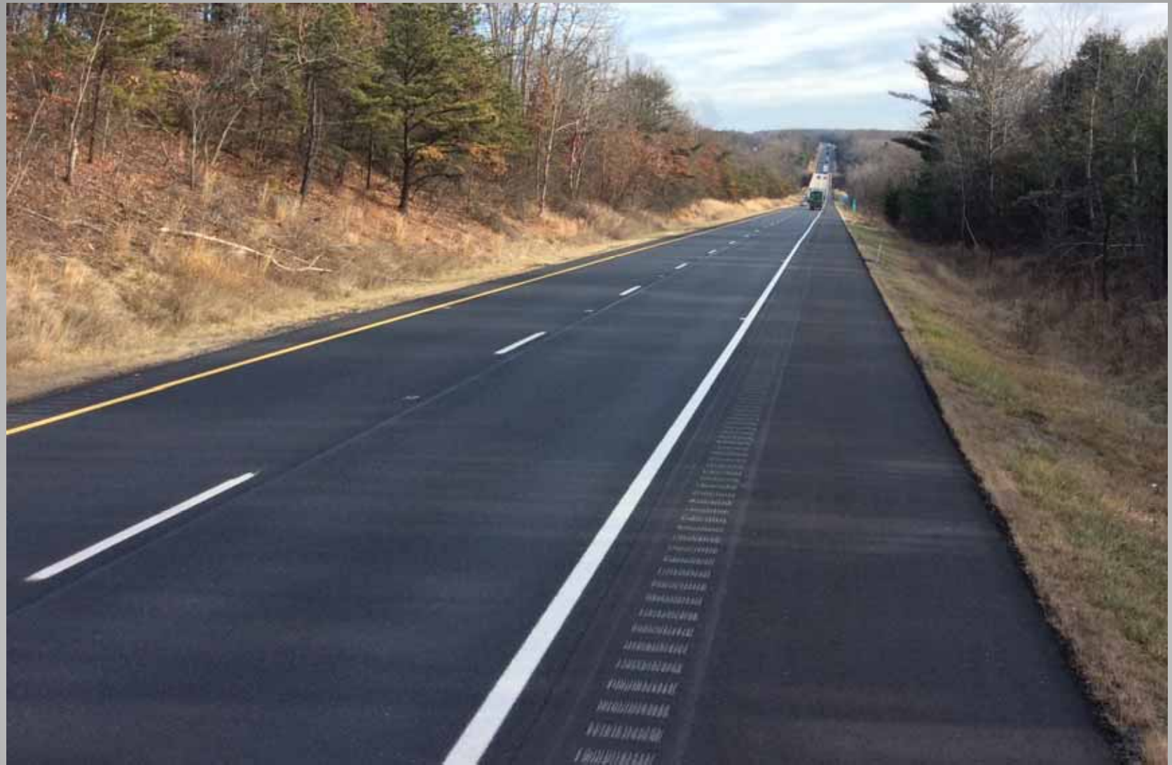
PennDOT District 5-0, The H&K Group
