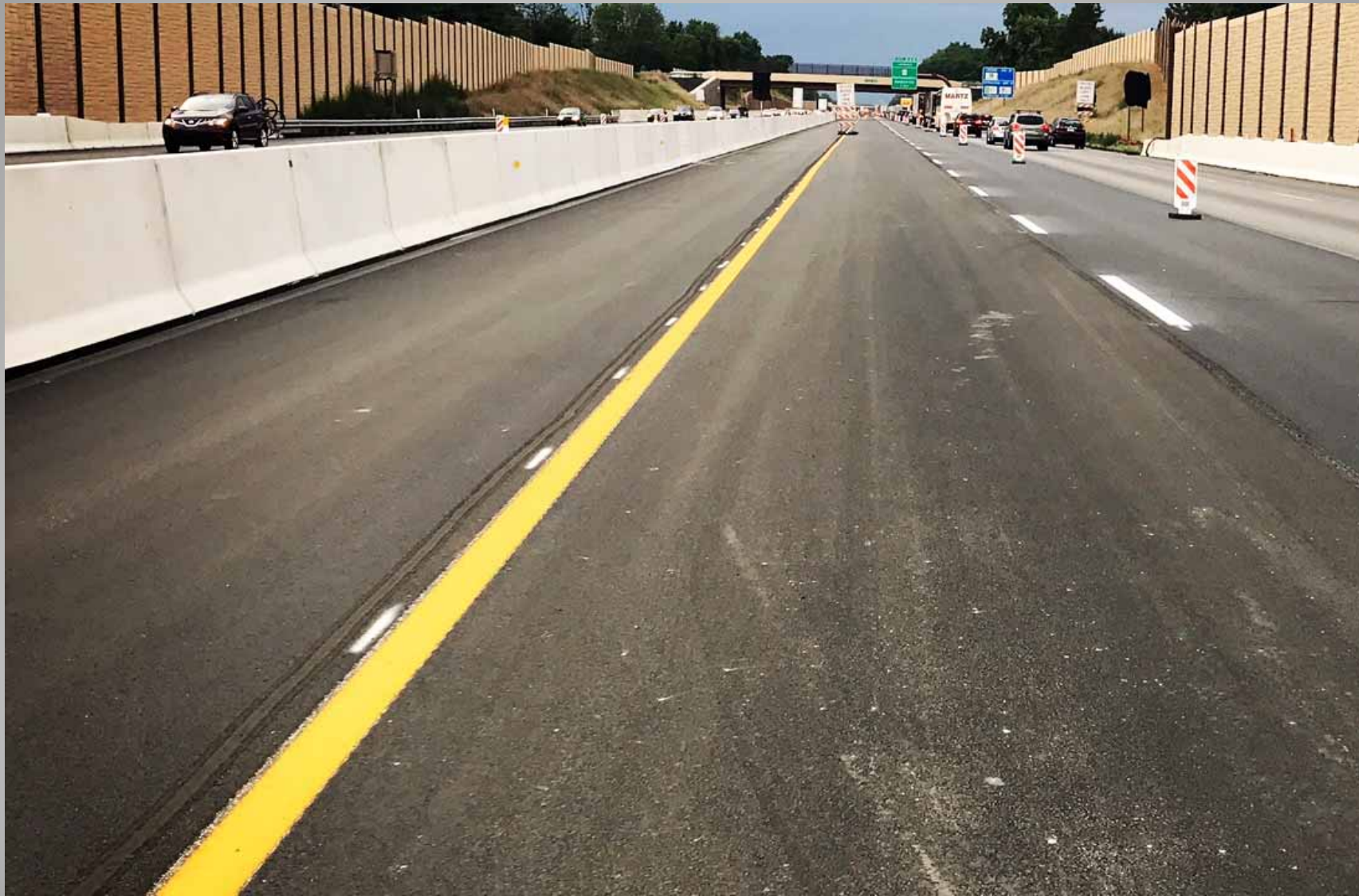
Pennsylvania Turnpike Commission, Allan Myers
