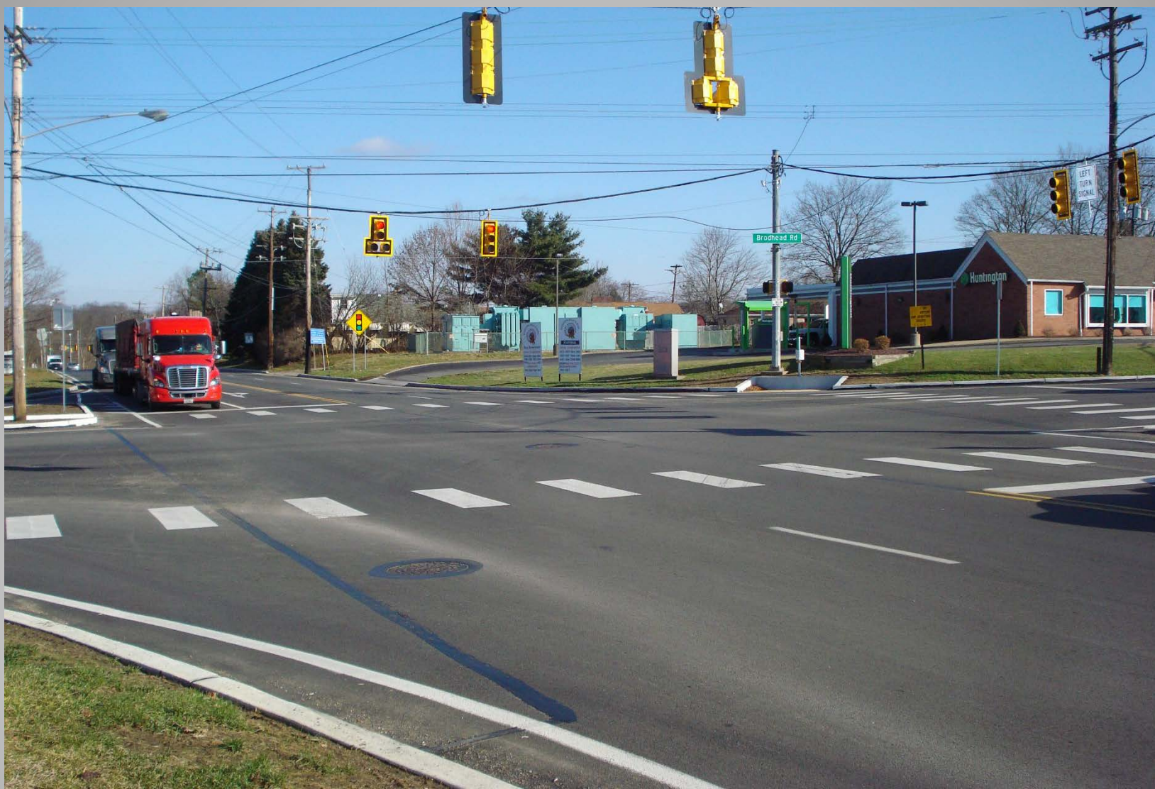
PennDOT District 11-0, Lindy Paving, Inc.
