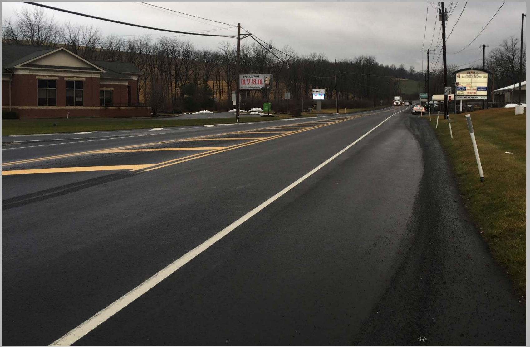
PennDOT District 5-0, The H&K Group
